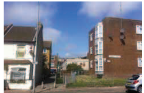
view to South site
